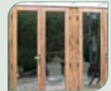
timber window frames
