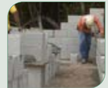
cement block walls
