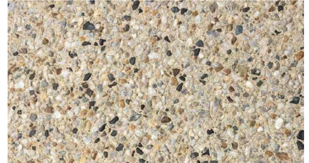
IN SITU CONCRETE PAVEMENT
