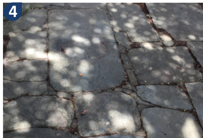
Slate flagstones - re laid to level and mortared
