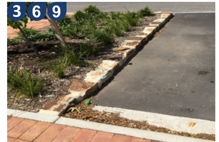
Bitumen to Carpark - Feature Stone Kerbing - Understorey Planting
