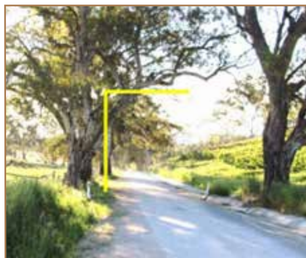
Figure 3.121 Clearance of vegetation within primary clearance envelope up to 6m high:
