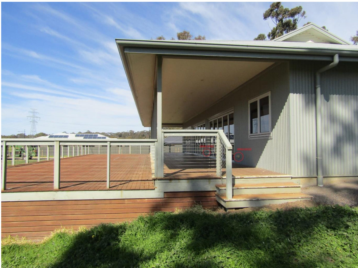
2 double GPOs on deck of Polo Grounds
