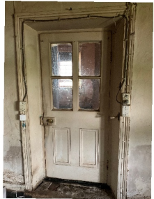
DOI-EXISTING INTERNAL DOOR SALVAGED FOR USE AS FRONT DOOR
