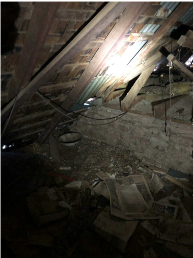
EXISTING PHOTOS OF EASTERN GABLE INSIDE ATTIC. PHOTO SHOWS THE VICTORIAN ADDITION TO BE DEMOLISHED AND SHOWS THE END OF THE TIMBER SHINGLE ROOF. THE NEW EASTERN GABLE END SHALL BE CONSTRUCTED ON TOP OF THE EXISTING STONE WALL AND MATCH THE EXISTING WESTERN GABLE END.
