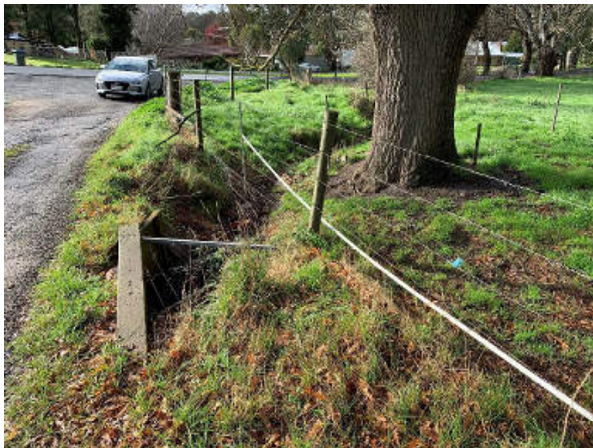
Tree 40 showing existing stormwater channel and culvert.
