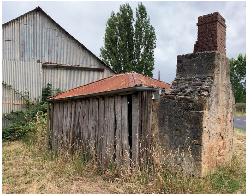
Figure 29 – Comparative example: early timber slab structure, Piccadilly.
