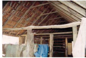
Interior of slab barn at Burnbank Farm (note shingle roof and tree-trunk frame), 1994
