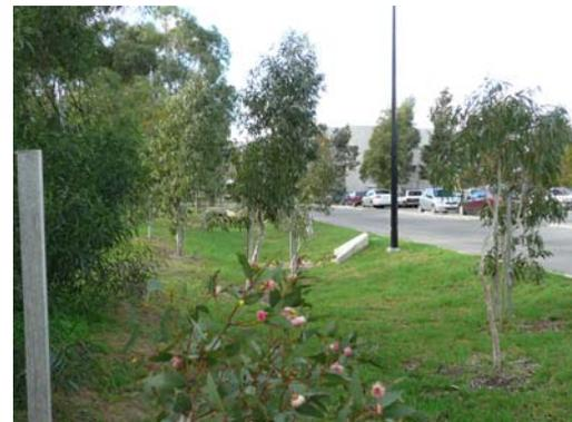
The street crossfall can be designed to fall towards an adjacent swale on one side of the street or towards the median strip. A swale may convey minor stormwater flows, whilst the carriageway itself is designed to convey major stormwater flows, as it would with a conventional kerb, gutter and pipe system.
