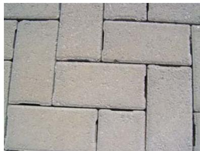
Benefits include reduced peak stormwater discharges, increased groundwater recharge, improved stormwater quality and multiple-use of paved areas.
